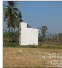
S7- Motor Room- 221m (SW)
