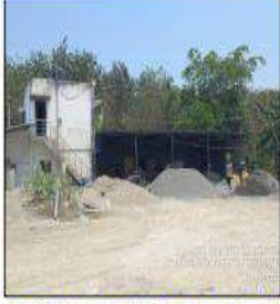
S1- Building Materials Shed- 96m (W)
