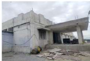
S1 – S4 Crusher Unit and its Office- 54m (S)
