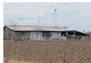
S10 – Farm shed - 297m (SE)
