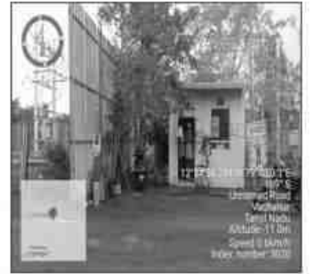
S8 – Security Cabin – 285m (E)
