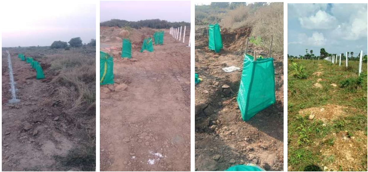
FIGURE 2.2: PHOTOGRAPHS OF GREENBELT & FENCING
