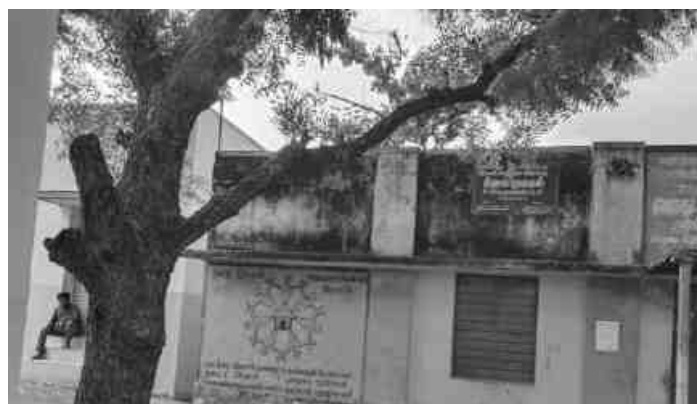
Sub Library, Appanayakkanpatti
