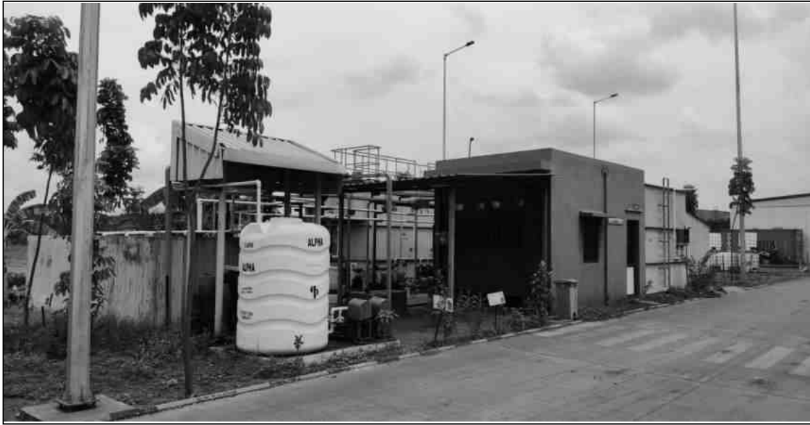
Figure 0.15. Images of STP & ETP
